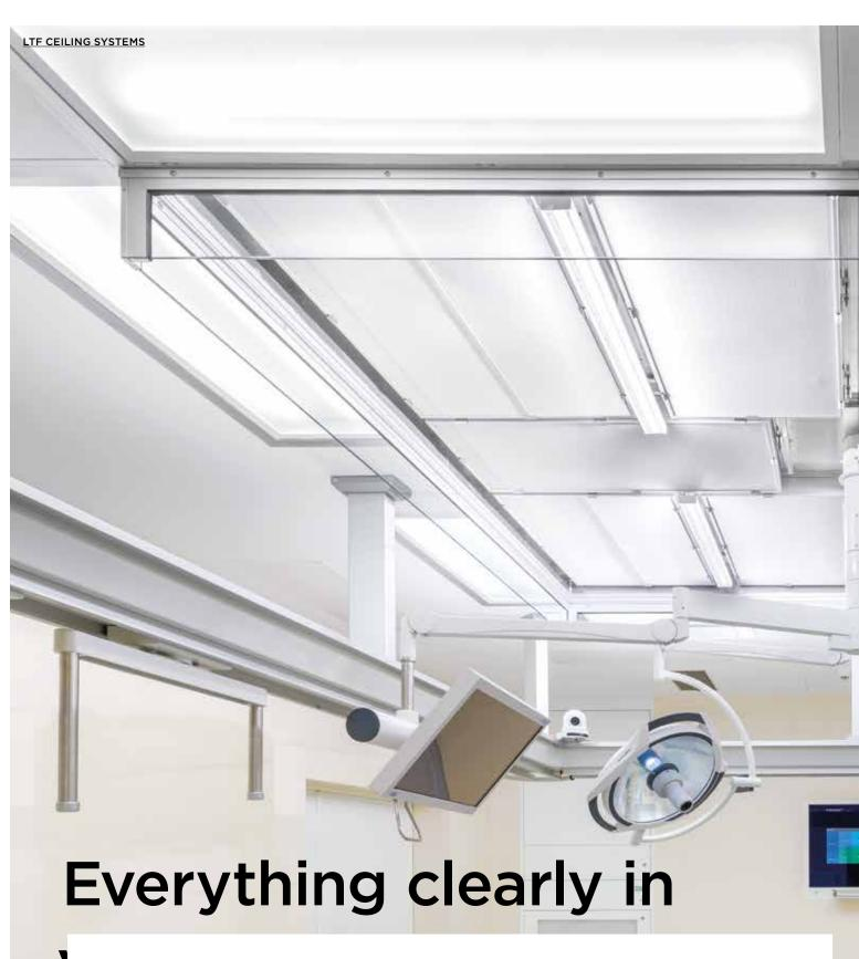
For most projects, integration of lighting into the LTF ceiling system is carried out as a result of increasingly individualised and specialised solutions of operating theatres. Due to the required different illumination levels, the common standards (EN 12464-1, DIN 5035-3) differentiate between operation field lighting, operation peripheral lighting and general lighting.
