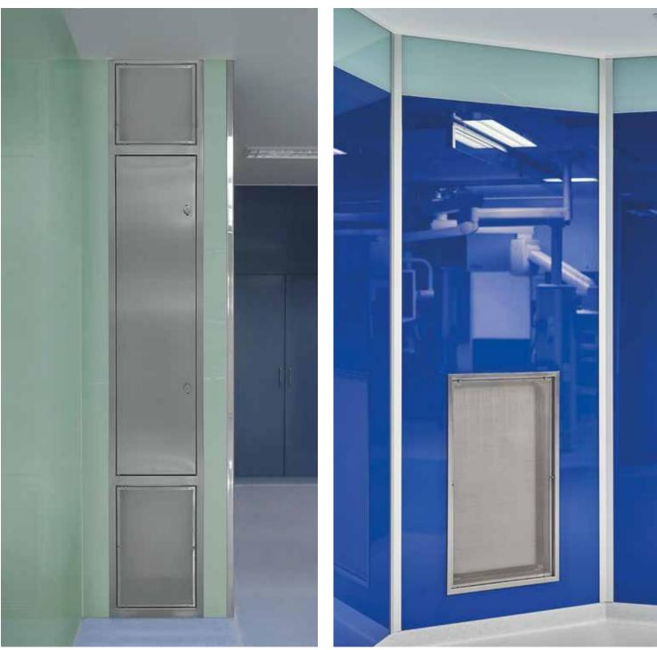
Exhaust air cabinet including fluff separator and inspection door
