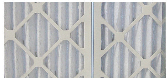
Gaps between standard cardboard pleated filter frames allow for air and particulate bypass
