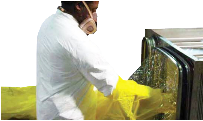
Fig. 9: Bag is resting on a parallel flat surface and not the floor
