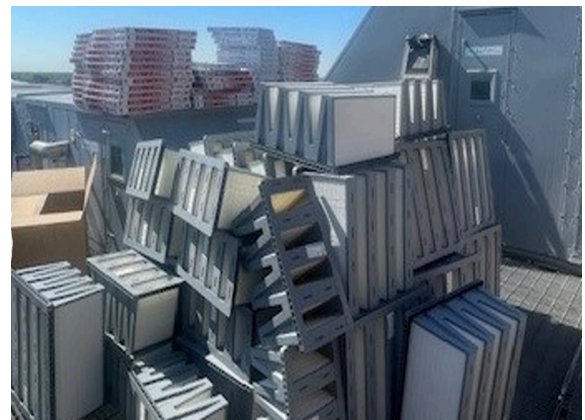
The MERV 16 V-Bank filters that were replaced
