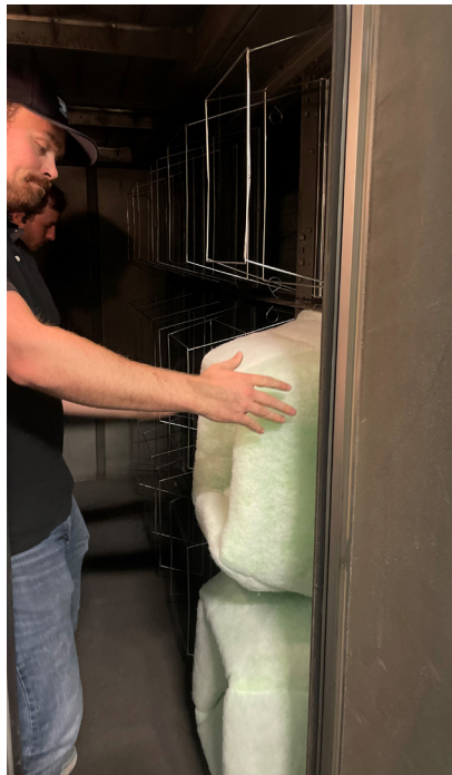
Installing the Tri-Cube RFX with center pocket on the retaining hardware
